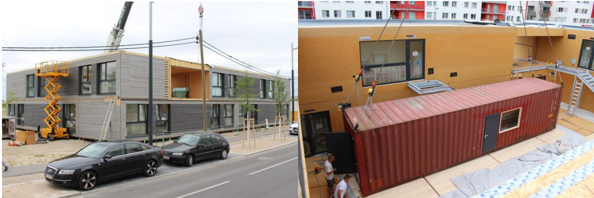
Picture 9+10 Mounting the PopUp GreenFlexStudios and the multifunctional container on the 6th working day
