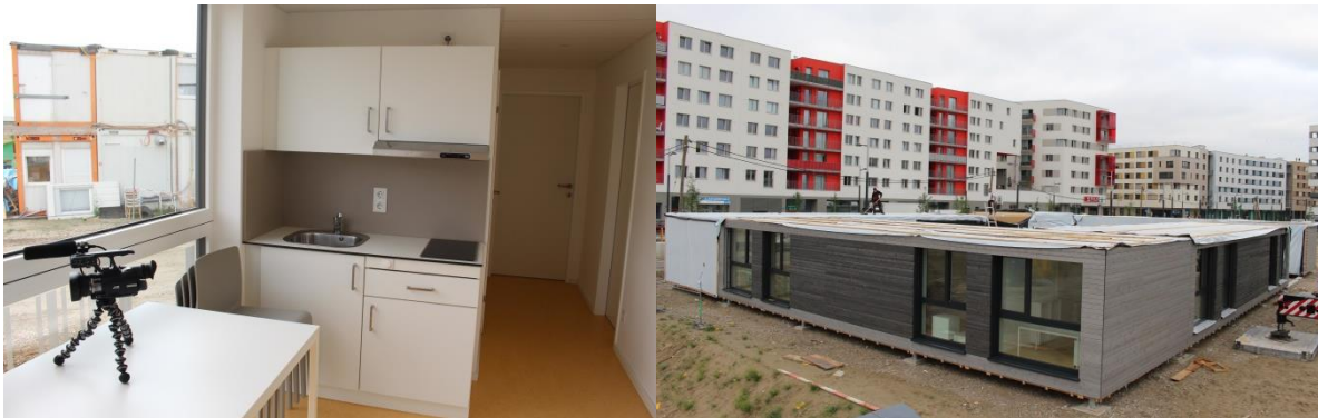
Picture 5+6 Fully furnished at delivery. Mounting the PopUp GreenFlexStudioBoxes on the 2 nd working day
