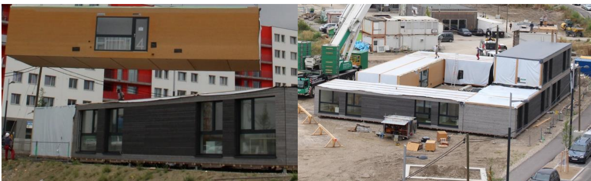
Picture 7+8 Mounting the GreenFlexStudioBoxes of the PopUp Dorms on the 2 nd working day
